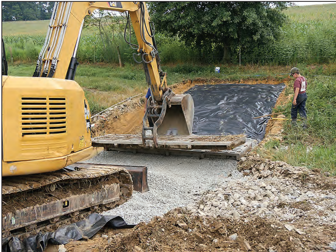
A stream crossing for cattle is installed on a farm in Lancaster County, PA. Financial aid from corporations increasingly is being funneled to farmers as consumers demand that products come from sustainable agriculture. (Maryland & Virginia Milk Producers Cooperative Association)
